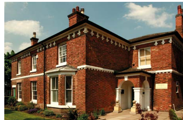
Rehabilitation houses in Burton
